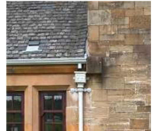
Original cast iron fittings at Glenfarg
