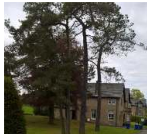
General view within conservation area
