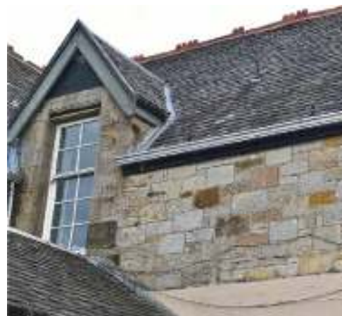
Replacement guttering in aluminium
