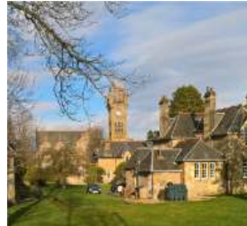
General view towards Mount Zion Church
