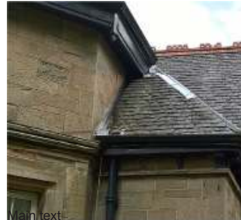
Overlaid zinc flashing over original lead
